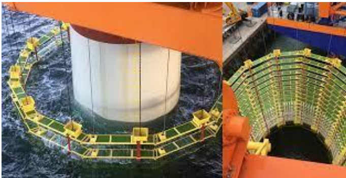
Deployment of near-field sound resonator: AdBm “coffee cups” filled with air around monopile
